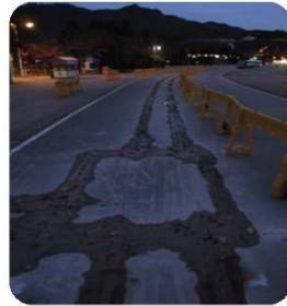
Cutting asphalt
