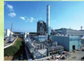
Demonstration facilities for oxygen-blown IGCC power generation (Osaki CoolGen Project)
