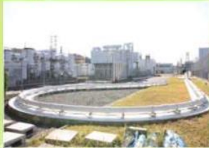
Superconducting cable system demonstration using actual grid
