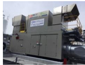
Hydrogen Gas Turbine (1.7MW)
